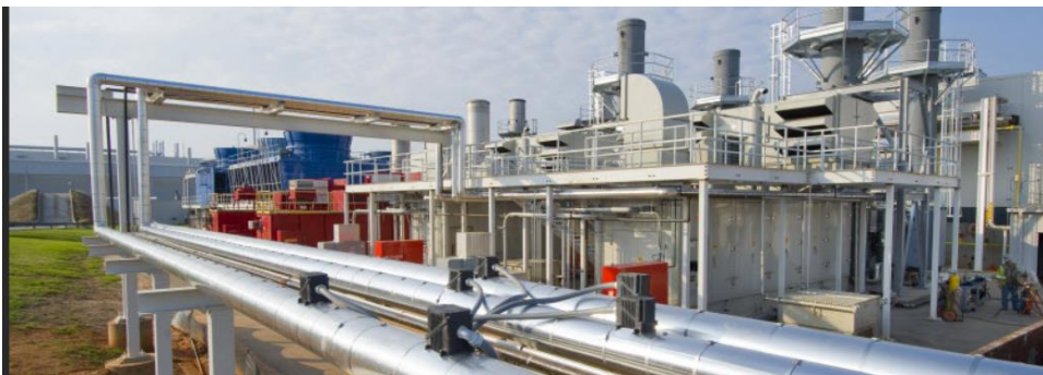
Figure 3. Above-ground pipe installation
